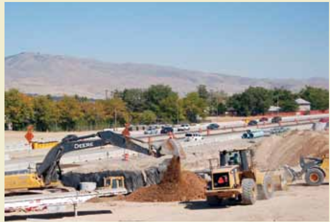
GARVEE funded I-84 project in Boise
